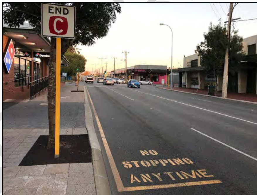
Finding 2.7 – End of Clearway and Line marking for No Stopping - easy to read and understand.
