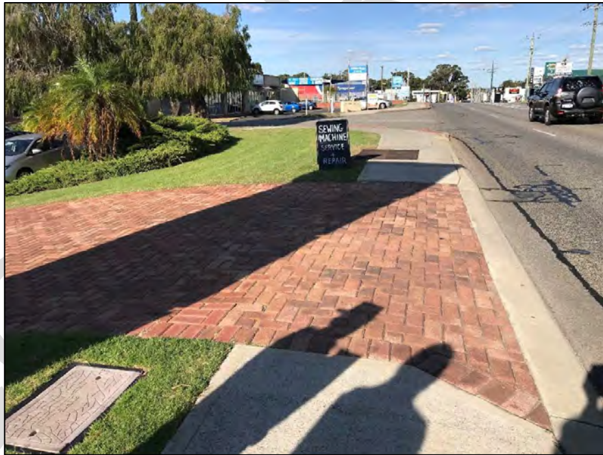
Finding 2.11 – Access constructed through the path.
