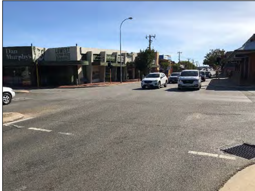
Finding 2.1 – Lack of central median along Pinjarra Road between the bridge and Sholl Street reduces the opportunity for pedestrians to cross the road safely.
