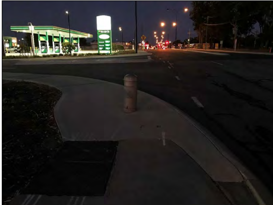
Finding 2.10 – A Telstra pillar in the path is difficult to see in dark conditions due to a lack of street lighting.
