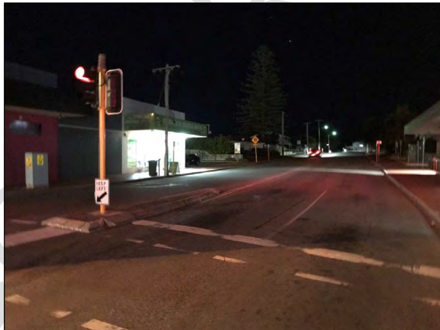
Finding 2.9 – Lack of street lighting on Lesley Street approaching the traffic control signals on Pinjarra Road.
