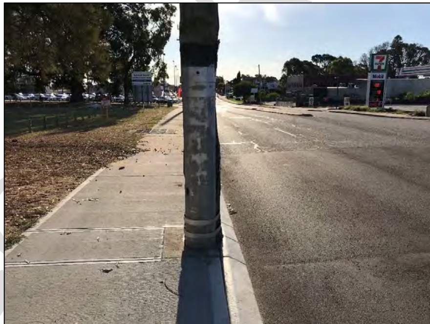
Finding 2.2 – Power Pole, which is not frangible within the Clear Zone is a hazard for errant vehicles.
