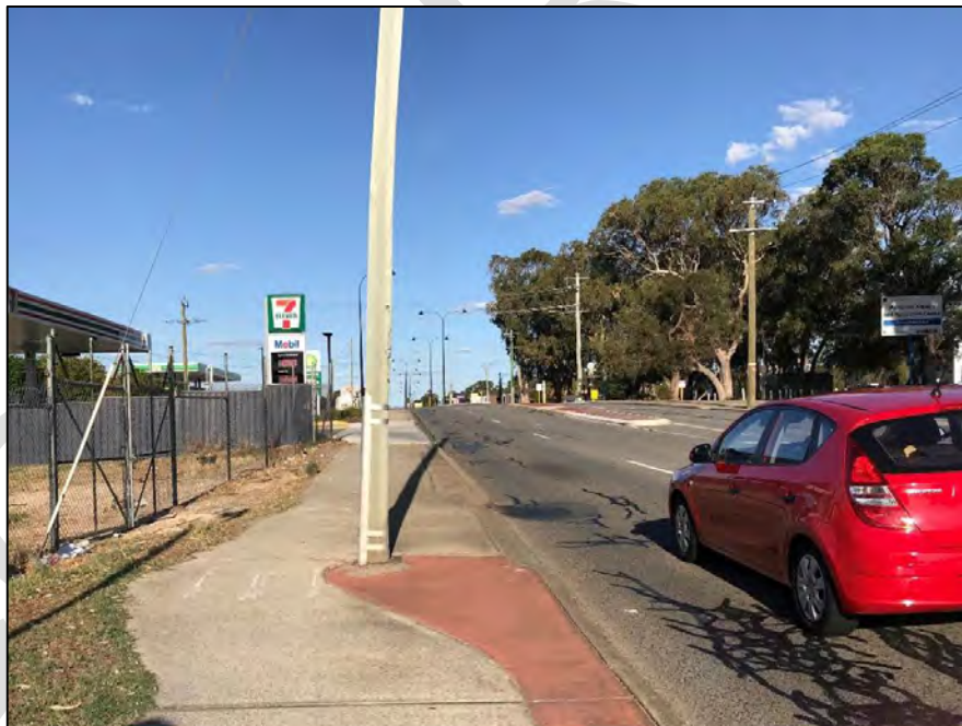
Finding 2.10 – Power pole in path with a contrasting colour used to assist guiding path users past the pole.
