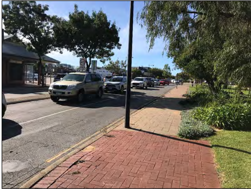
Finding 2.11 – Path of different widths and paving material.
