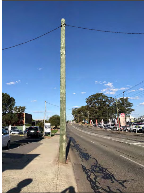
Finding 2.2 – Opportunity to place the power service underground enabling the removal of the pole, or the pole could be relocated into private property.
