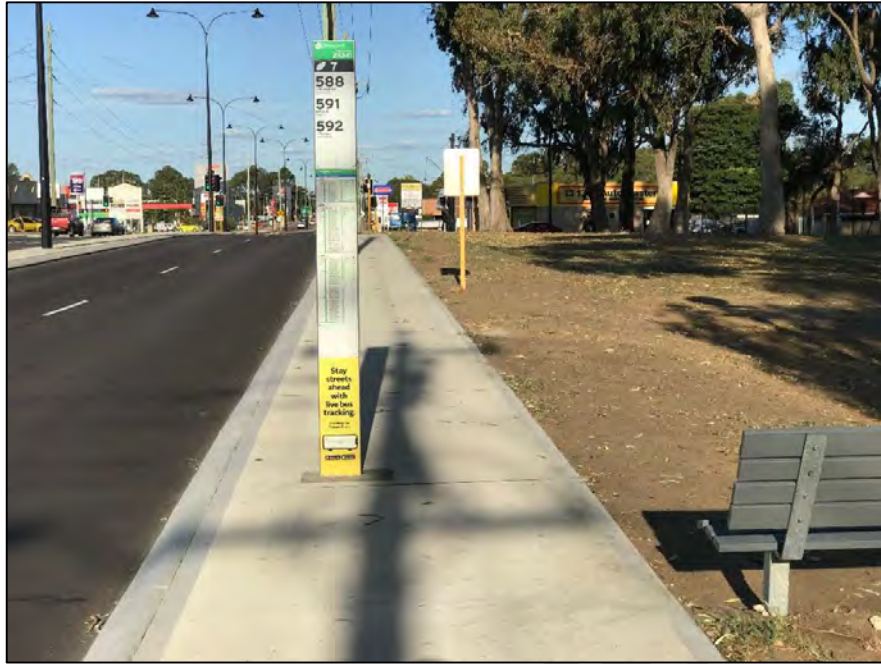
Finding 2.10 – Bus information post is an obstruction in the path.
